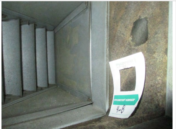
Photo 22: Sample # 4-8: VAV 4-11: Rm 225B Isolation vibration material, LP side; MSFV= 21403, Category II Aspergillus/Penicillium and Chaetomium
