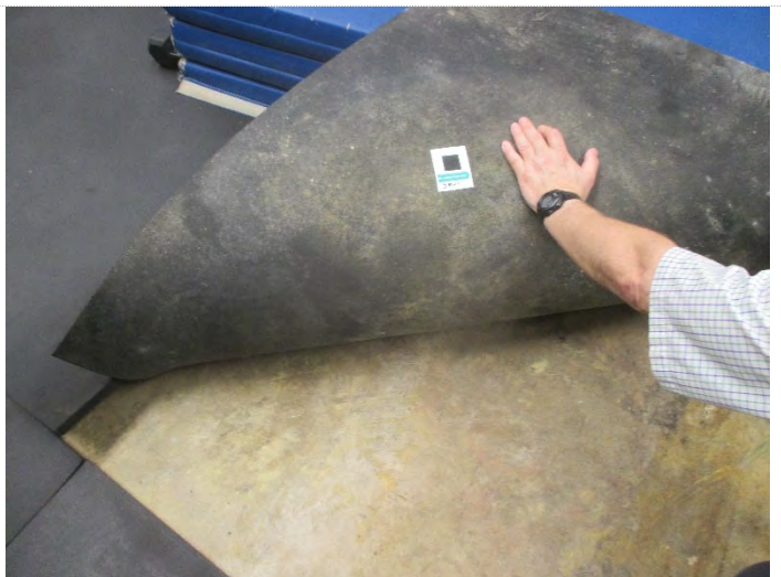
Photo 40: Sample # GM-1: Gym floor mat backside surface, Mat #4 from left MSFV= 6077 Category II Vegetative mold growth (Asp/Pen-like) due to moisture through slab or water damage from flooding reported, Mat # 4 from left- facing emergency exit door
