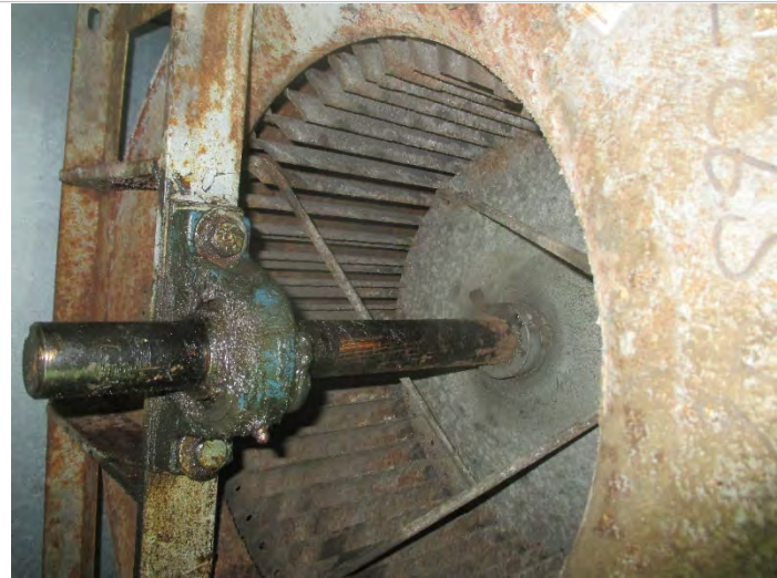
Photo 11: Sample # 3-1: AHU-3 Fan blade, far side MSFV= 2726, Heavy debris with evidence of over greased bearings
