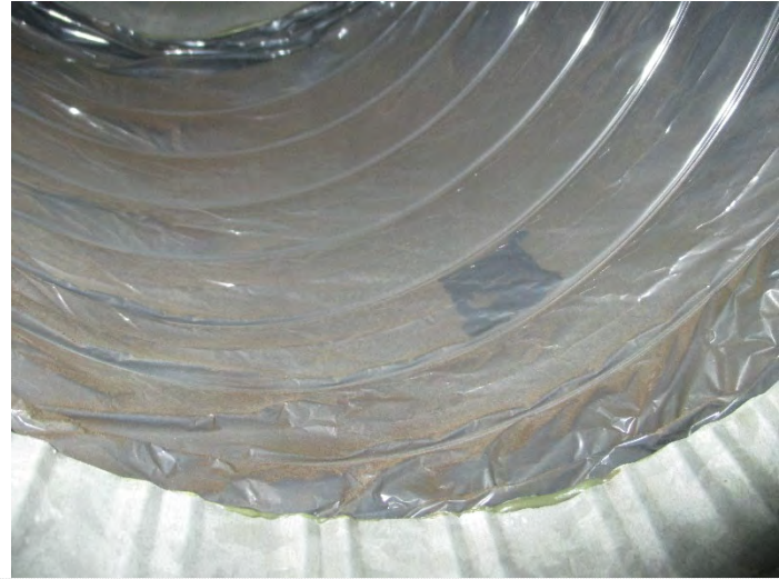
Photo 15: Sample # 3-10: VAV F3-3: Rm 108 Flex supply duct; MSFV= 6046
