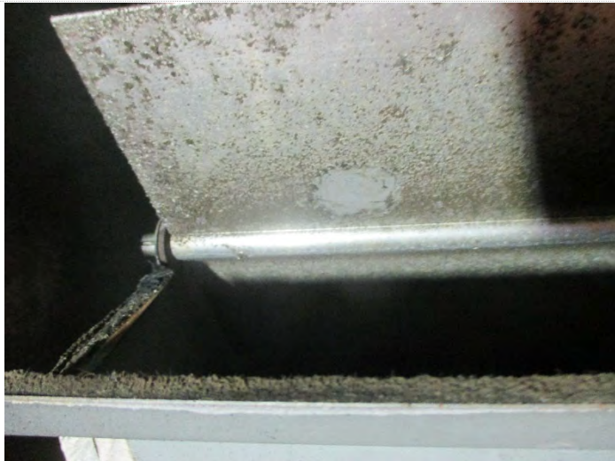
Photo 3: Sample # 1-5: VAV F1-1 Damper MSFV= 4312, Heavy debris, located in hallway floor near Rm B008
