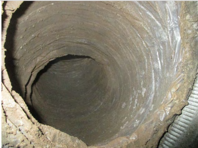
Photo 18: Sample # 4-3: Mechanical room flex duct from main supply trunk, MSFV= 10519
