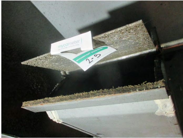
Photo 7: Sample # 2-5: VAV F2-2, Hallway damper, near Rm 108; MSFV= 6971
