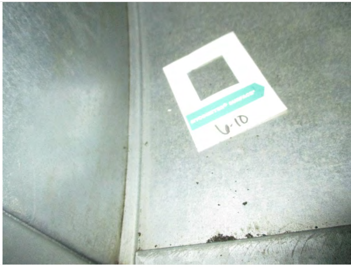
Photo 36: Sample # 6-10: Rm 442E LP Metal supply duct MSFV= 40
