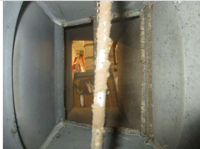
Photo 27: Sample # 5-5: Reheat unit, inlet side of heating coils, MSFV= 4384, Category IV Acremonium Mold Growth (Excessive debris on coils of re-heat) before cleaning
