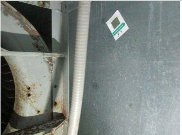
Photo 12: Sample # 3-4: AHU-3 Side panel with grease deposits, MSFV= 5
