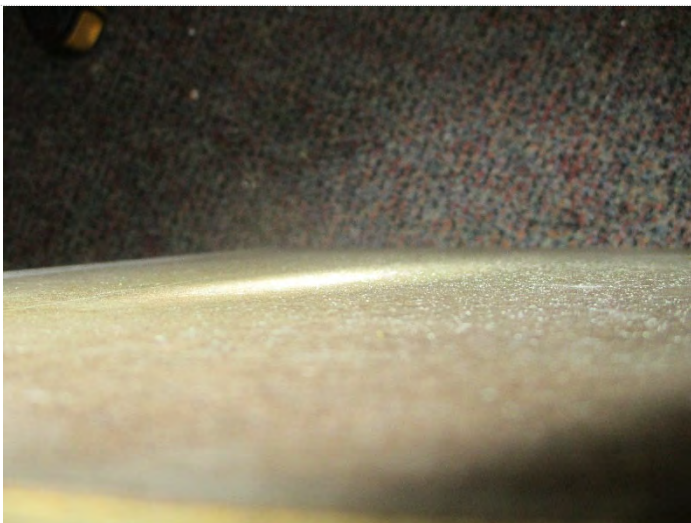
Photo 39: Sample # 420-3: Room 420 Built-in bookshelf, Underside (bottom); Category IV Mold Growth of Aspergillus and Penicillium
