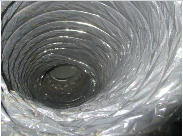
Photo 28: Sample # 5-6: Rm 326 Supply flex duct MSFV= 898, "Cleared"
