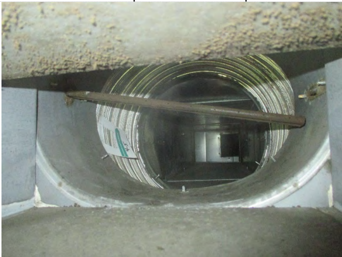
Photo 19: Sample # 4-5: VAV 4-11, Rm 225B Flex thermo fin, upstream of HP; MSFV= 2312, Mold Growth Category IV Aspergillus/Penicillium on internal metal surface of Thermo fin flexible duct
