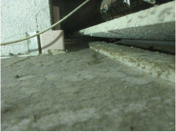
Photo 10: Sample # 2-10: Dust from the top of the ceiling tile near VAV F2-2; Category IV Mold growth of Penicillium/Aspergillus and Cladosporium Growth in Dust Deposits
