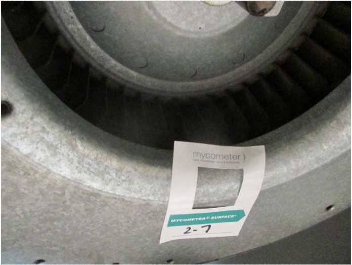
Photo 8: Sample # 2-7: VAV F2-2, Fan blade, near Rm 108; MSFV= 145
