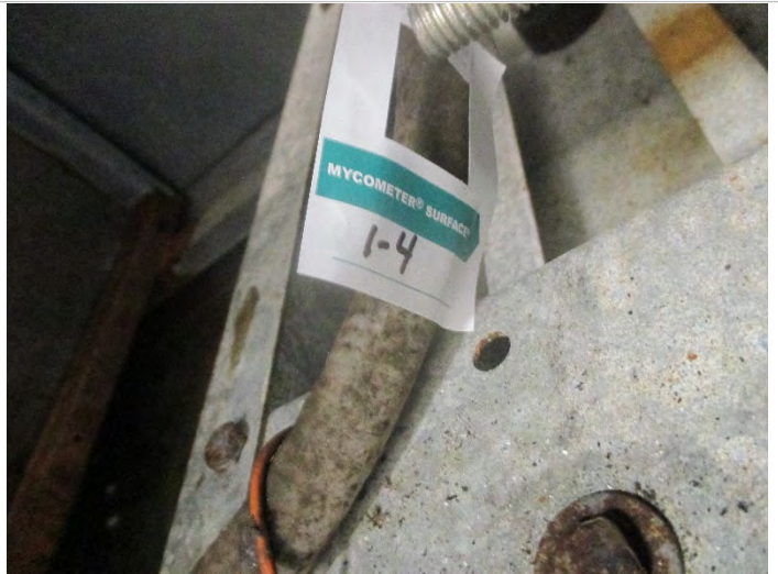
Photo 2: Sample # 1-4: AHU-1 Power line to blow motor, MSFV= 7903; Category IV Aspergillus/Penicillium on plastic coating of electrical cable inside AHU
