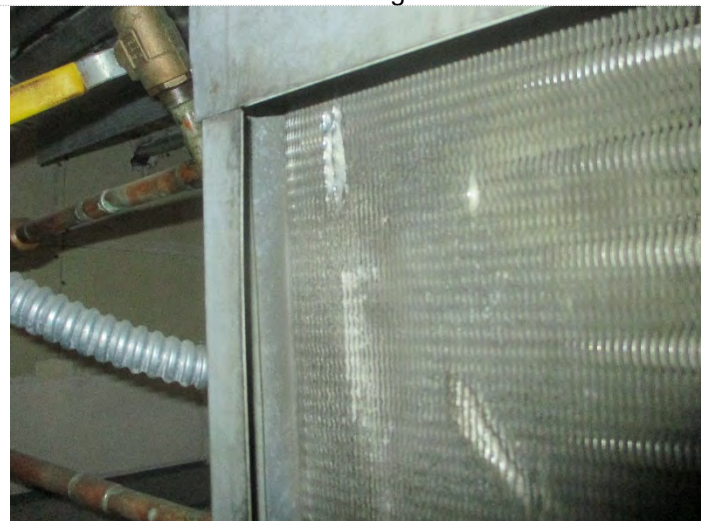
Photo 29: Sample # 5-8 Rm 318 VAV Cooling unit, inlet MSFV= 33, Dirty, had to bend filter to move it
