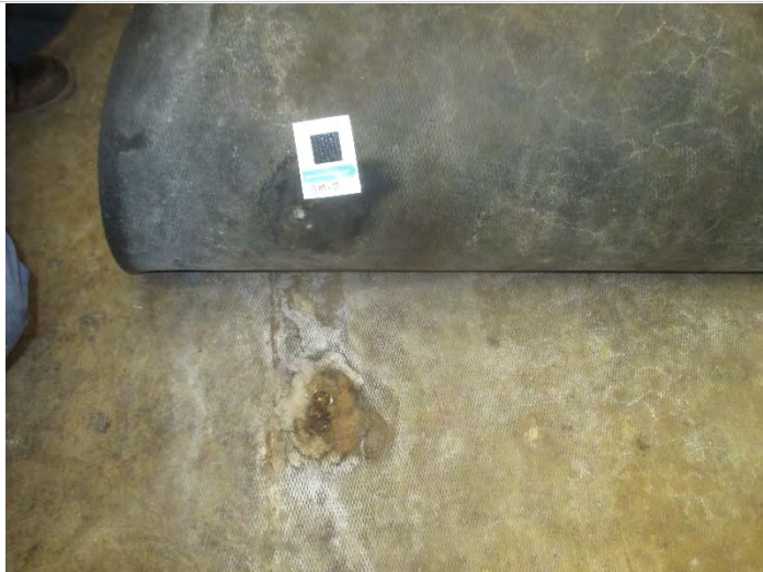
Photo 41: Sample # GM-2: Gym floor mat backside surface, Mat 14 from left MSFV= 7731 Category II Vegetative mold growth (Asp/Pen-like) due to moisture through slab or water damage from flooding reported, Mat # 1 from left-facing emergency exit door
