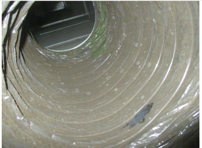
Photo 4: Sample # 1-8: VAV F1-1 HP Flex supply duct MSFV= 2086, Located in hallway floor near Rm B008
