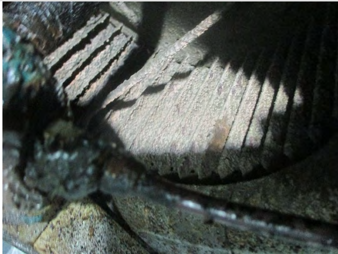
Photo 1: Sample # 1-2: AHU-1 Fan blade, far side MSFV= 5179; over greased bearings with heavy debris
