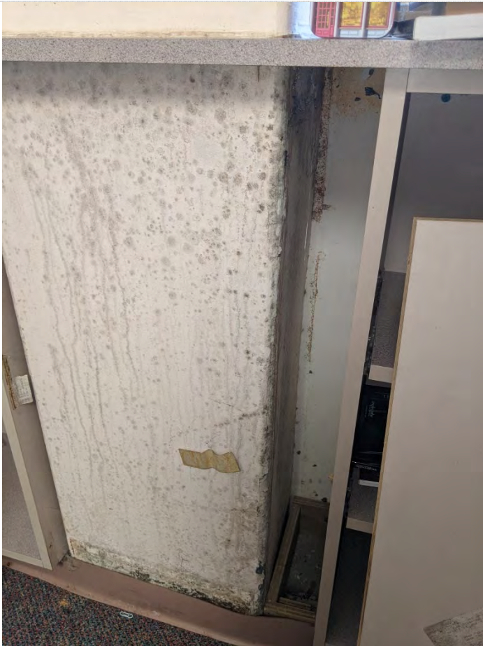
Photo 37: Sample # 220-1: Room 220 Column built-in bookshelf, front; Category II Low density mold growth of Aspergillus/Penicillium and Cladosporium
