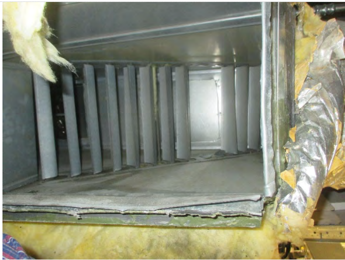
Photo 35: Sample # 6-6: Reheat Unit C6-6 LP Metal Supply Duct pass Rm 440 VAV; MSFV= 35, Category IV Old, inactive mold growth Cladosporium
