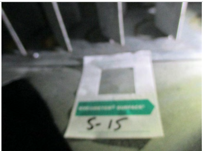
Photo 32: Sample # 5-15 Corner hallway base of HP supply duct, near turning vein; MSFV=30, Near stairway stairs
