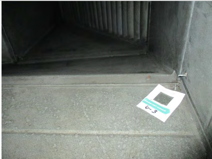
Photo 33: Sample # 6-3: AHU-6 HP supply duct plenum; MSFV= 16
