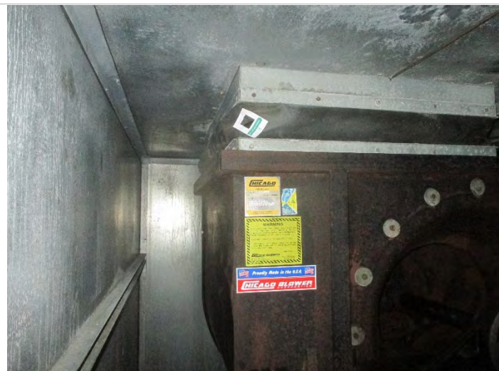
Photo 25: Sample # 5-3: AHU-5 Isolation vibration material, MSFV= 136, SMG
