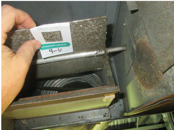
Photo 20: Sample # 4-6: VAV 4-11, Rm 225B Damper MSFV= 10944, Heavy debris and Mold Growth Category IV Cladosporium with moderate deposits of Aspergillus/Penicillium
