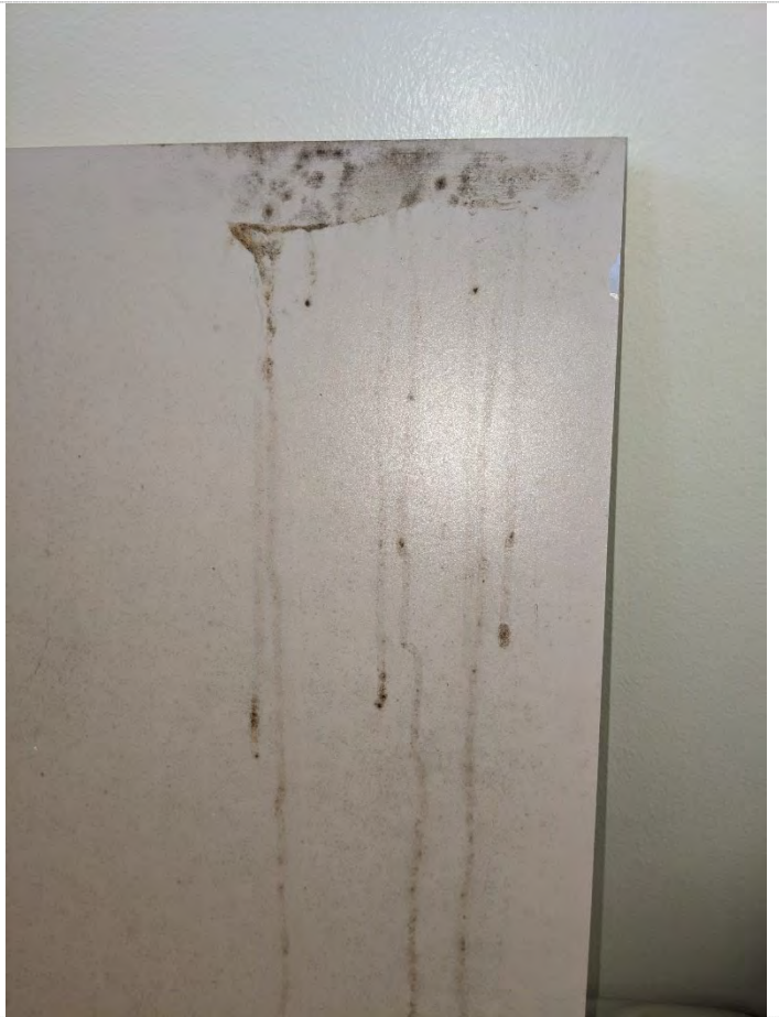
Photo 38: Sample # 328-3: Room 328 Built-in Bookshelf, Back Cover Category IV Mold Growth of Cladosporium
