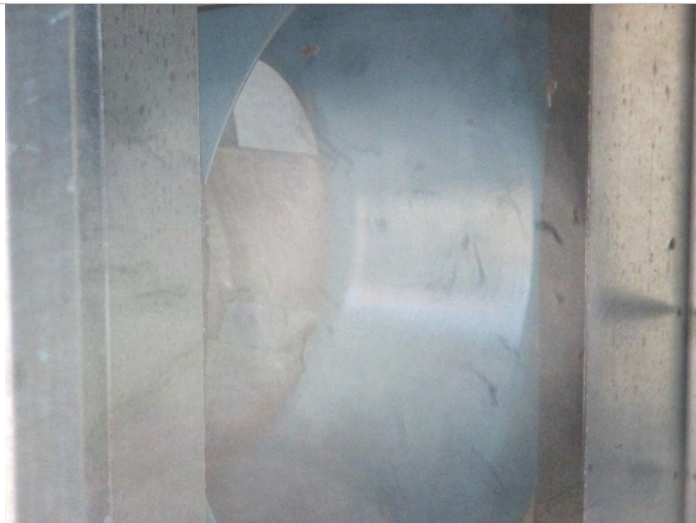
Photo 43: Sample # RT-2: Rooftop AHU Fan blade MSFV= 4, Access from 411 Mech Rm
