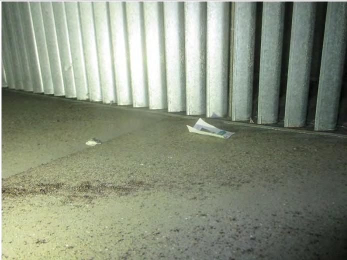
Photo 17: Sample # 4-2: Main supply trunk, access hatch near mechanical room entrance, MSFV= 797, Deposited mold growth shed from fan; Category III Cladosporium and Pen/Asp
