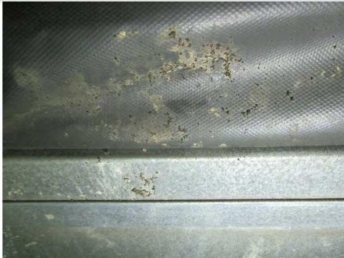
Photo 5: Sample # 1-9: VAV F1-1 LP Isolation vibration material MSFV= 185, Located in hallway floor near Rm B008
