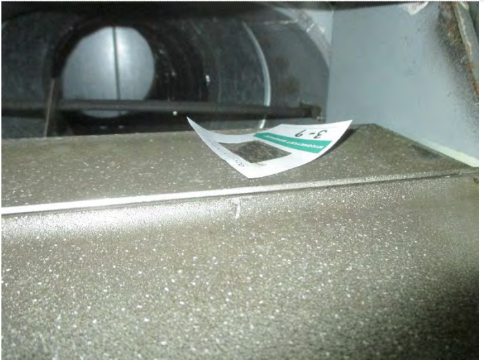
Photo 14: Sample # 3-9: VAV F3-3: Rm 108 Damper; MSFV= 12037
