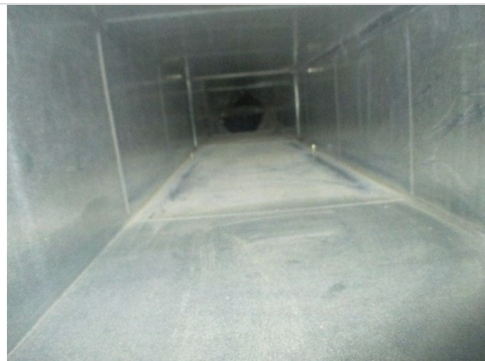
Photo 31: Sample # 5-14 Rm 332C LP Metal supply duct MSFV=45
