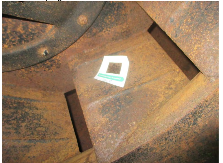
Photo 22: Sample # 4-8: VAV 4-11: Rm 225B Isolation vibration material, LP side; MSFV= 21403, Category II Aspergillus/Penicillium and Chaetomium
