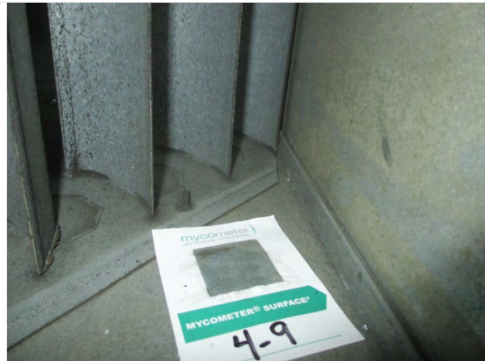
Photo 23: Sample # 4-9: VAV 4-11: Rm 225 Metal supply duct; MSFV= 145; Category II Aspergillus/Penicillium and Alternaria
