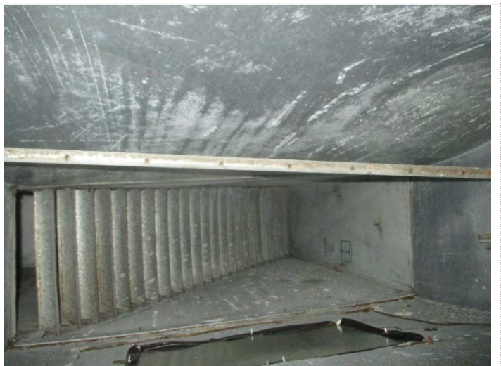
Photo 26: Sample # 5-4: AHU-5 Supply outlet turning vein, MSFV= 148, In Mech. Room
