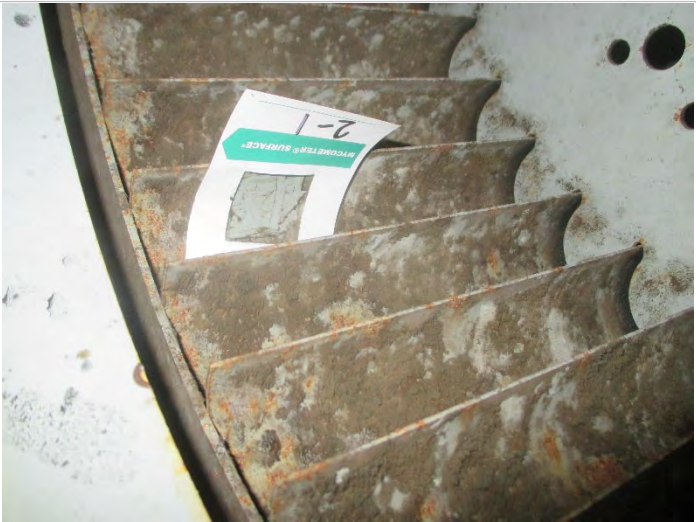
Photo 6: Sample # 2-1: AHU-2 Fan blade, far side MSFV= 7211
