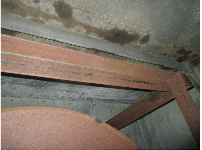
Photo 16: Sample # 4-1: AHU-4 Supply chamber outlet, top wall; MSFV= 322, (2nd floor) Above blower wheel
