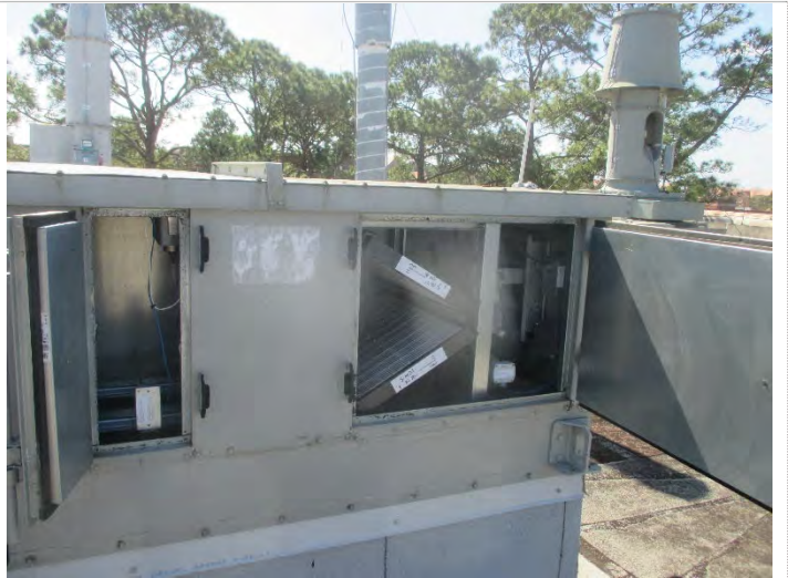
Photo 42: Sample # RT-1: Rooftop AHU cooling coils inlet MSFV= 0, Access from 411 Mech Rm
