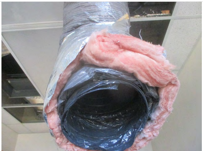
Photo 30: Sample # 5-11 Rm 316 Flex supply duct outlet MSFV= 184
